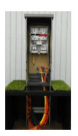
The cabinet should be installed to measure at least 850 mm above ground level.
