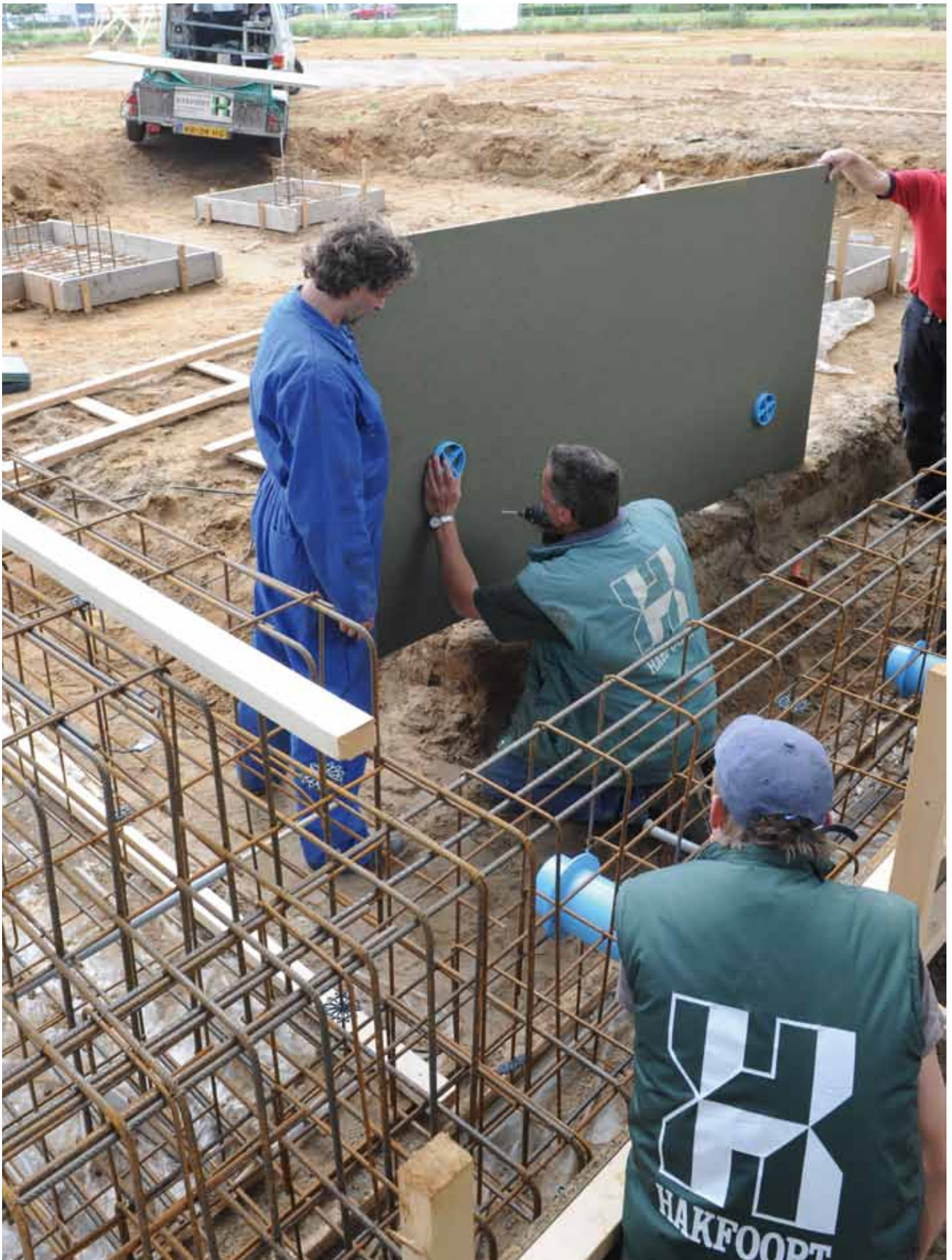
The fixation pieces of both conduits are fixed to the casing plate.
