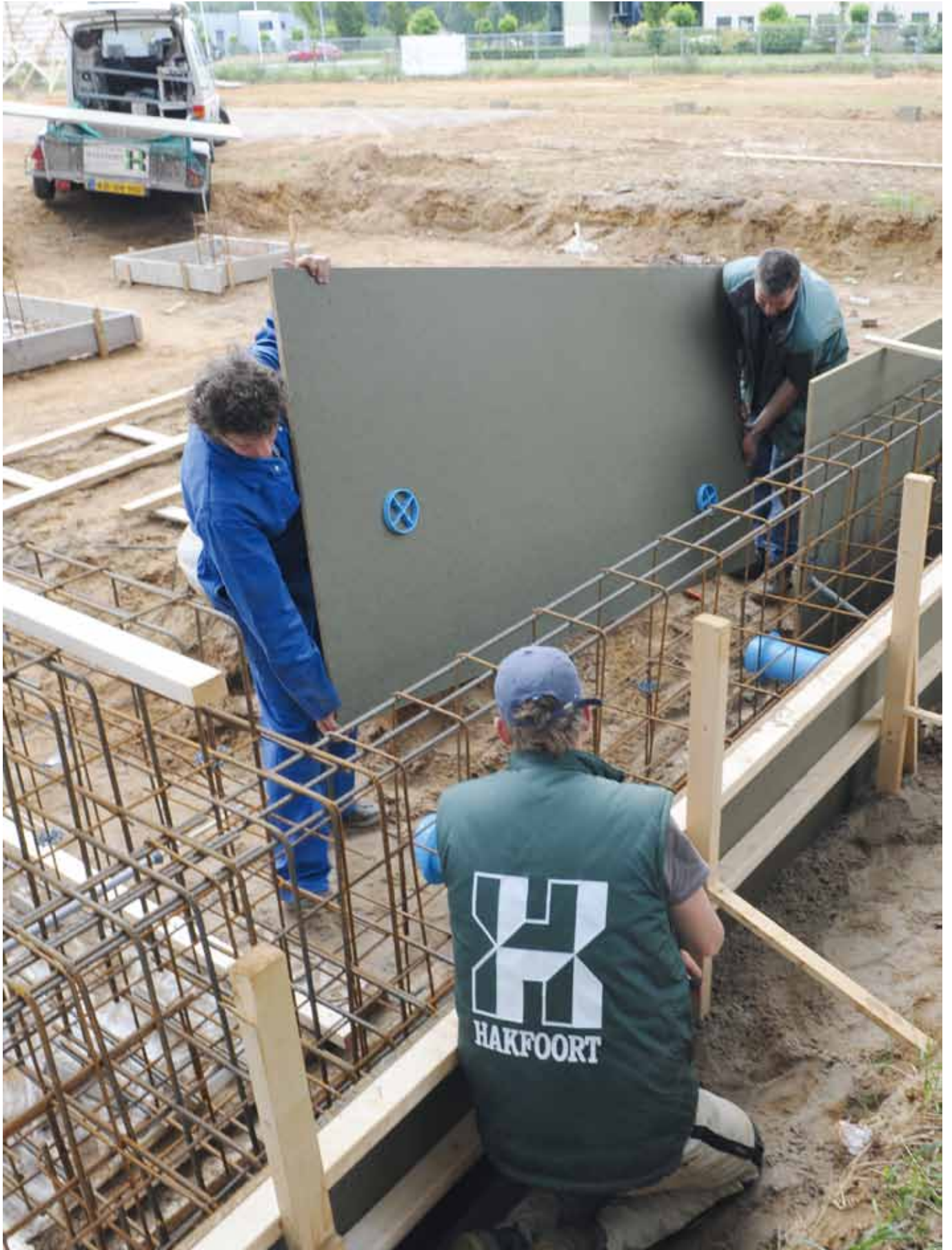
Casing plate placed back on its position.
