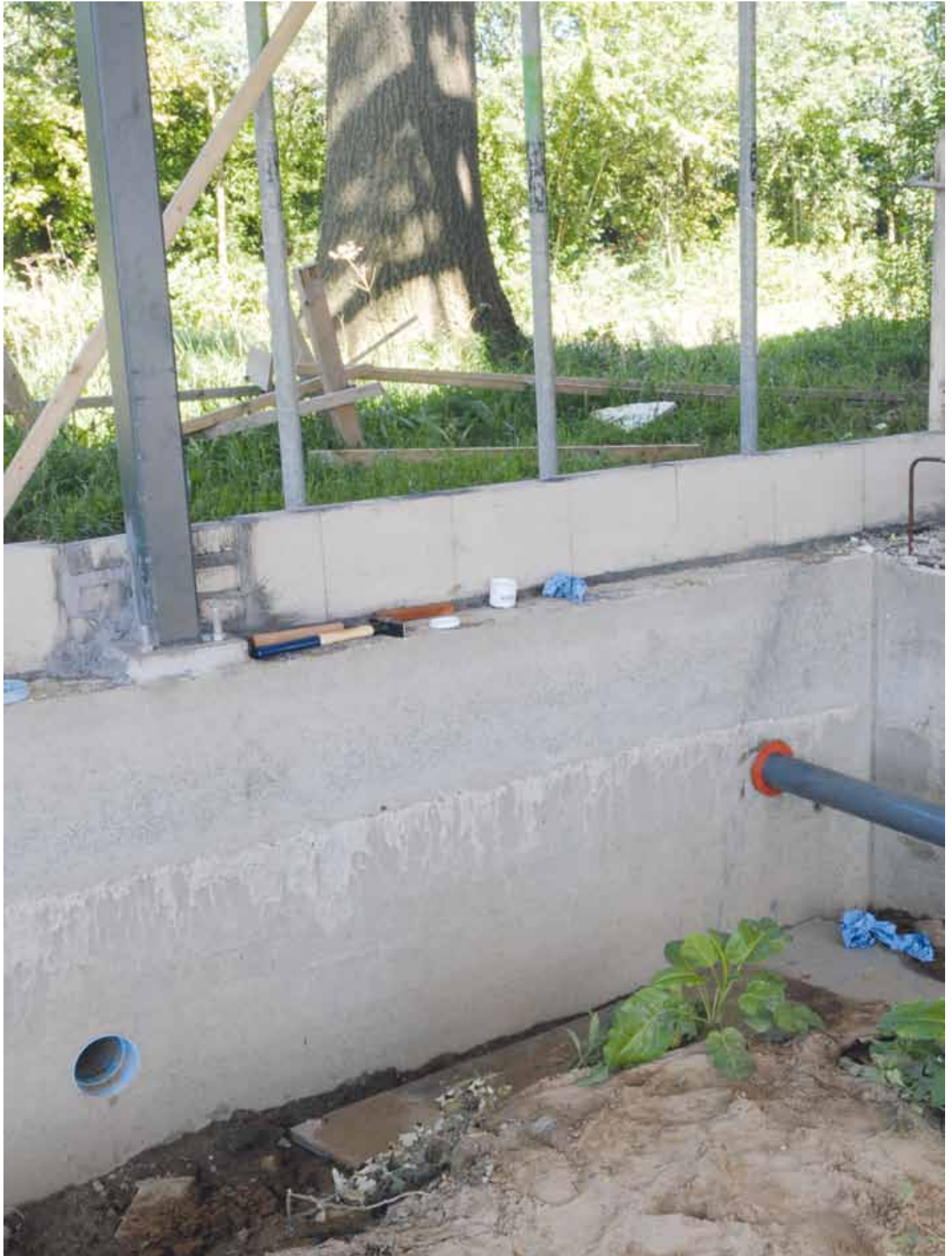
Situation in the construction.
