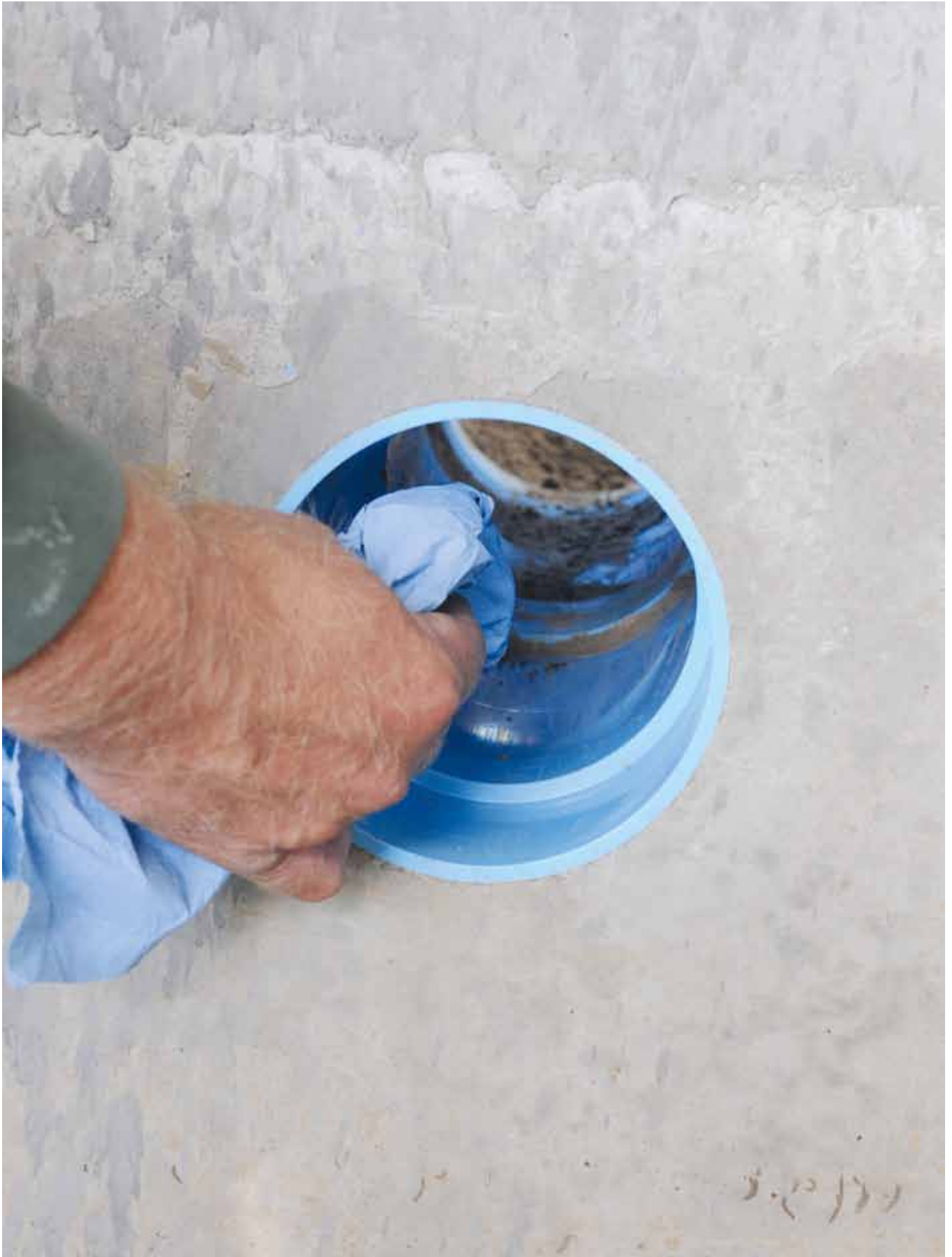
Cleaning the inside of the conduit inlet.
