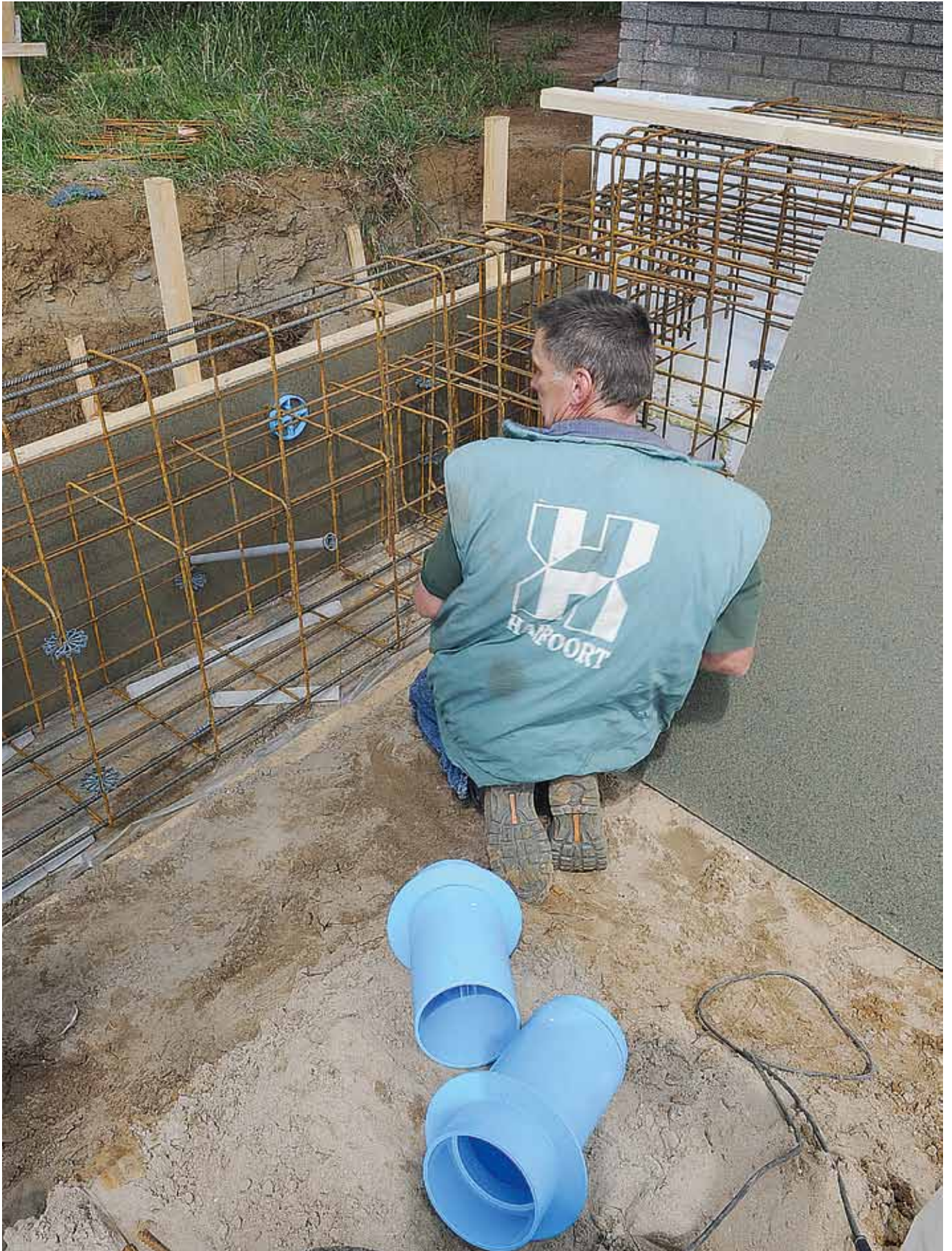
The conduit inlet system set has been prepared to fit into the casing. A conduit inlet with an adapter pipe with standard length (200 mm). In the front a conduit inlet, adapter pipe cut to size and a connector.
