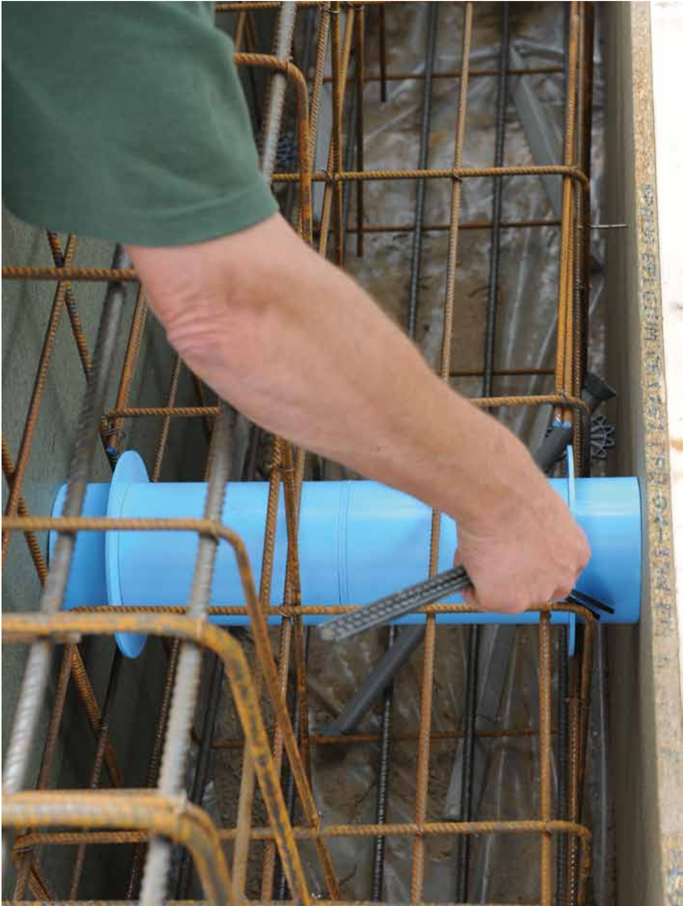
The building supervisor, using the CSD® embedded conduit inlet system for the first time, was excited about it and especially liked the distance from the flange to the casing plate.
