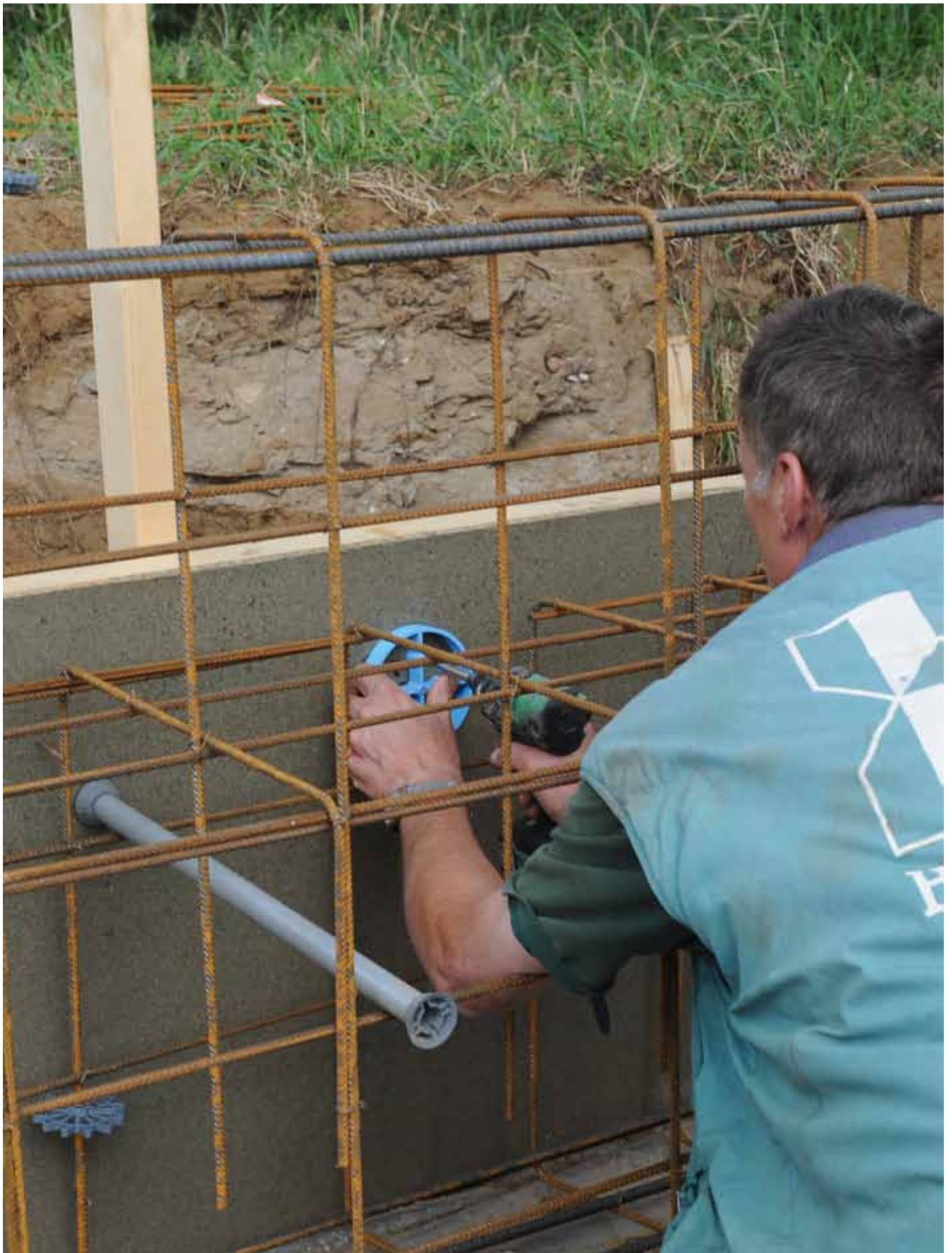
The fixation piece of the CSD® embedded conduit inlet system is fixed onto the plating.
