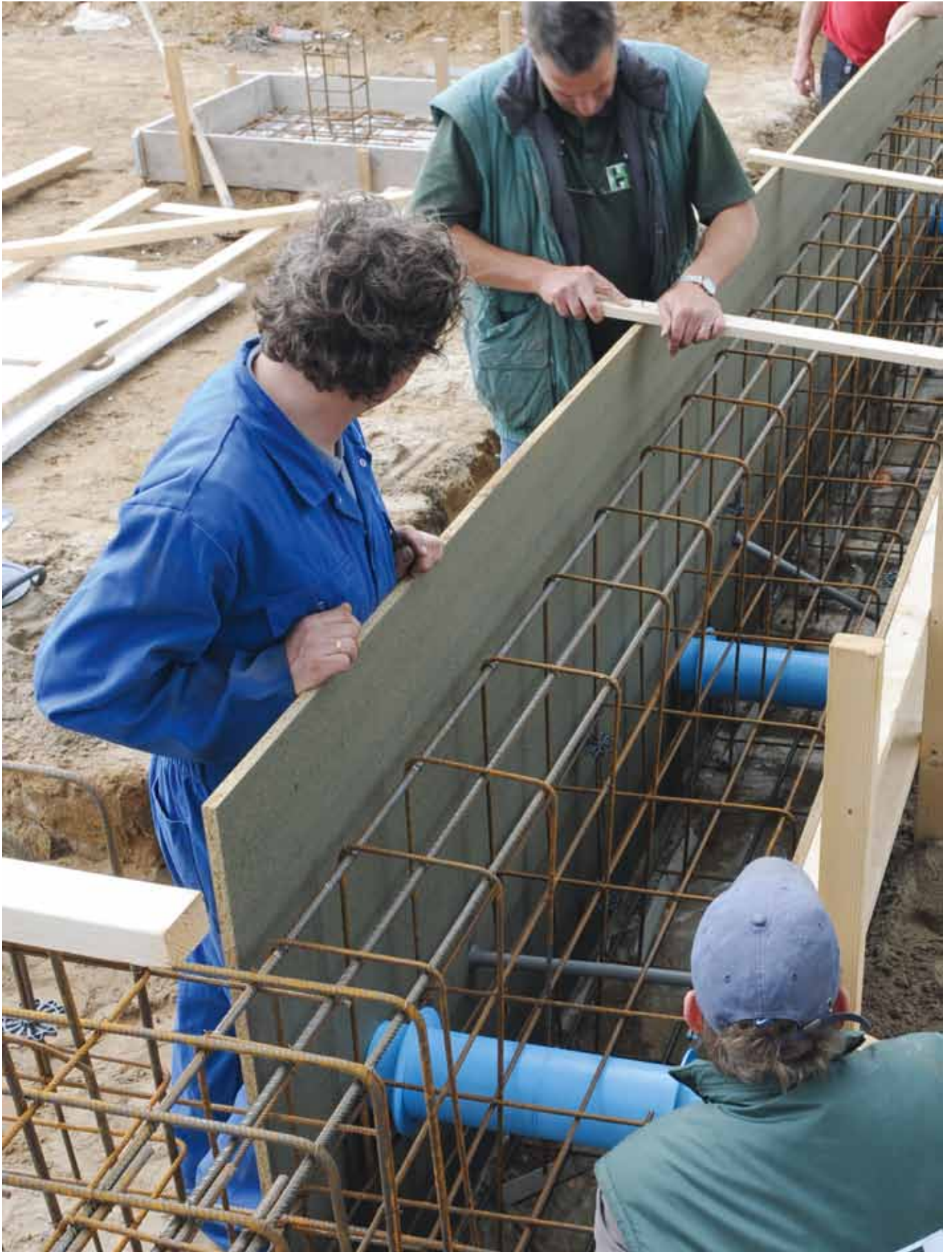
Casing plate is provisory fixed for further finishing of the casing .
