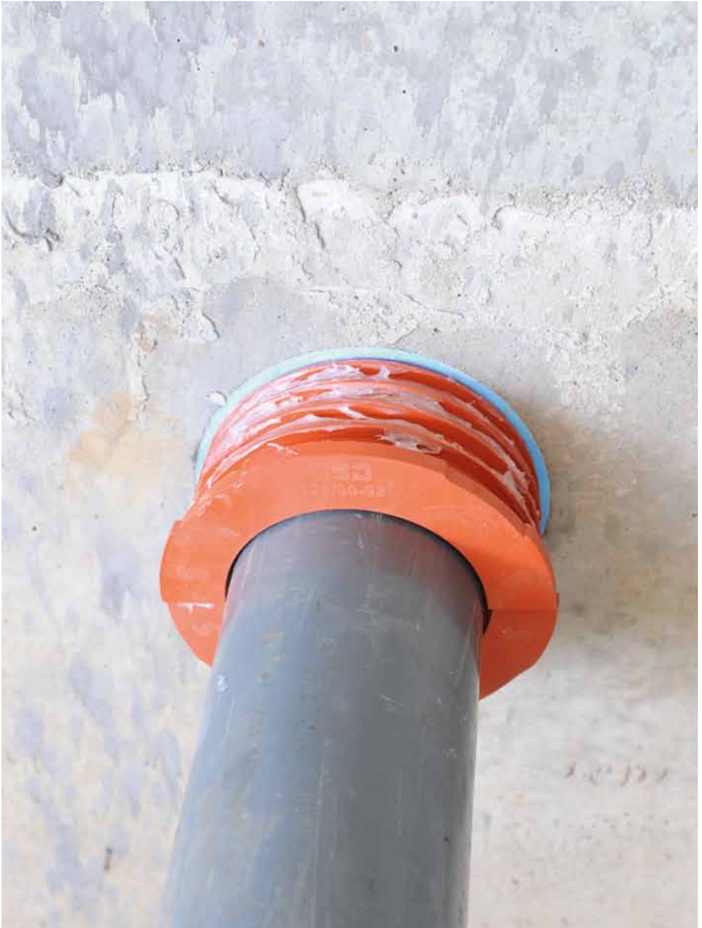
SLIPSIL® plug 125/90-92 lubricated and inserted over the first serration into the CSD® conduit inlet.
