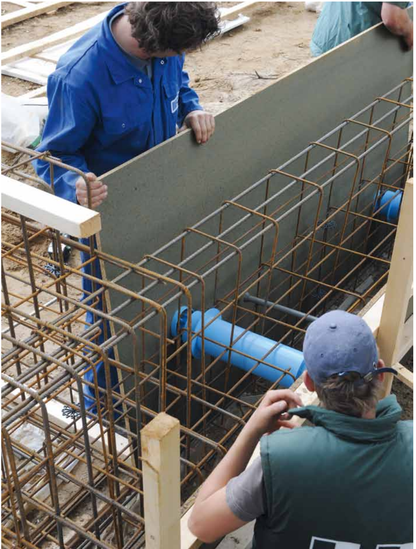
The fixation pieces are pushed into the conduit inlets.
